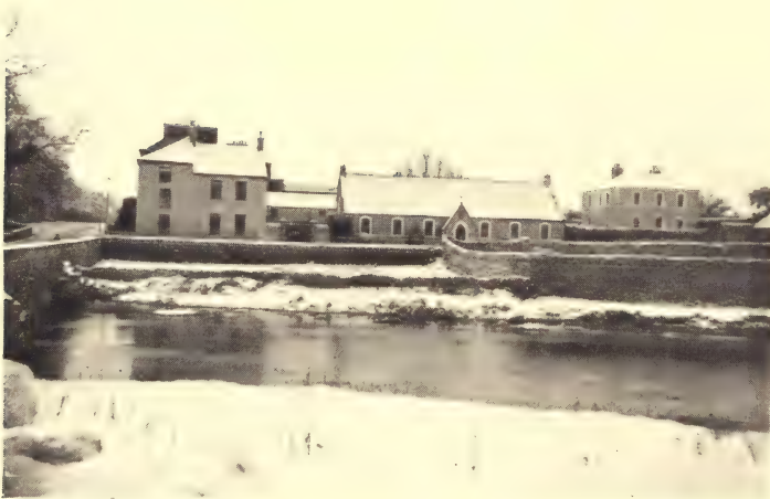
"BRIDGE HOUSE" AND BOYS' SCHOOL, DONERAILE
